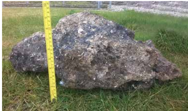
Fatberg pulled from a burst 6 inch sewer in Cambridgeshire
