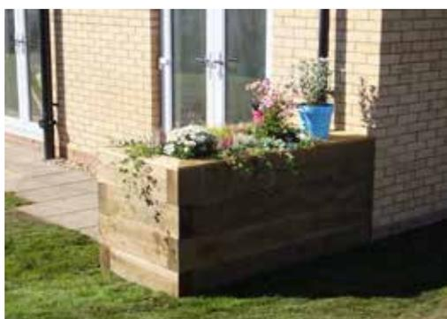
Raised bed raingarden, Taylor Wimpey show-house (courtesy B J D'Arcy). Raised bed raingarden units with free-draining soil need plants able to cope with wet or dry conditions.
