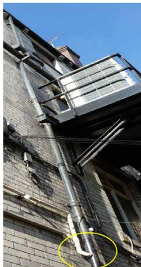
Neat job but clearly a misconnection into roof drainage
