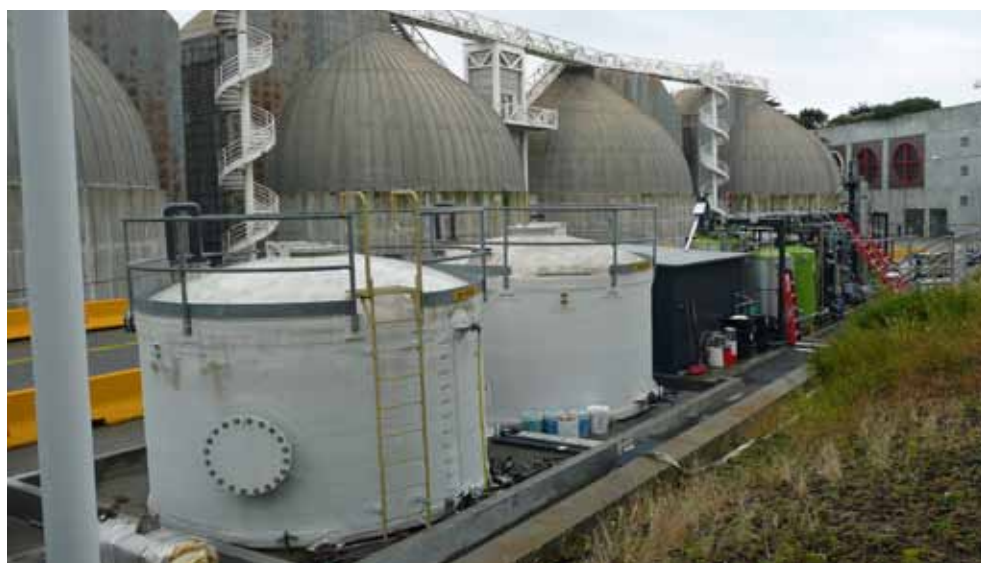
The FOG to biodiesel pilot plant at Oceanside WwTW with the digesters in the background.
